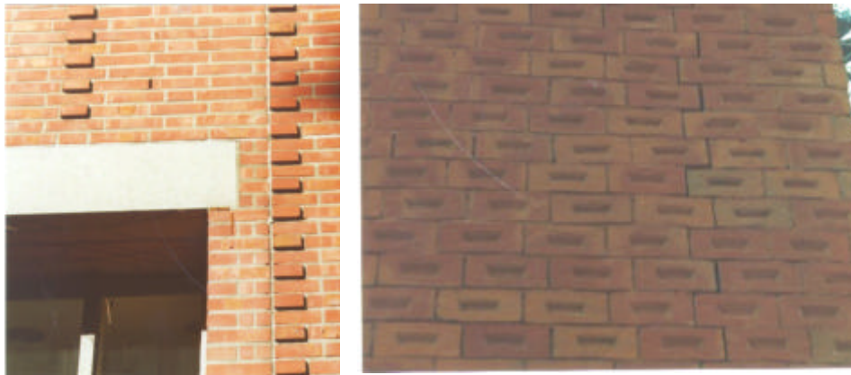
Figure 3 Two types of movement joints
