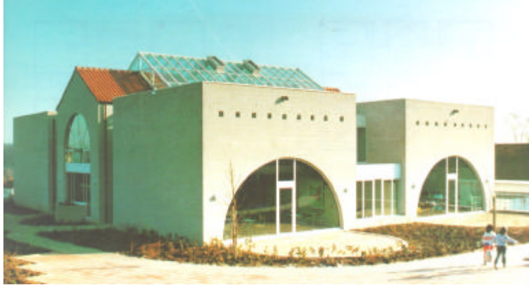
Figure 10 Example of recessed walls, wall high windows and arches
