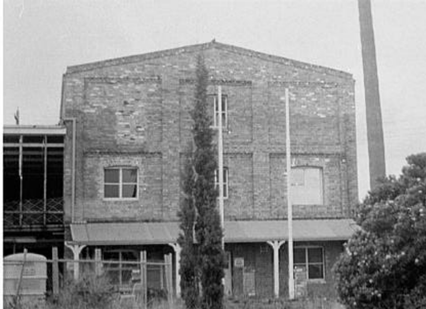
Figure 7. Flour Mill after repairs from the damage of the 1989 Newcastle Event.
