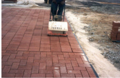
Vibration of Stack Bond, Area #1 Figure 4
