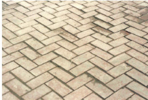
Figure 10 Movement of Pavers, Ohio December 1992
