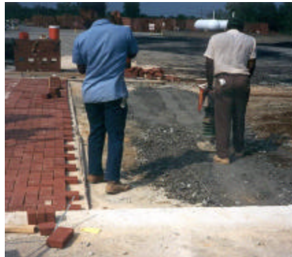
Compaction of Base, Area #1
