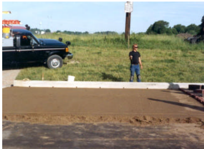
Installation of Setting Bed Figure 5
