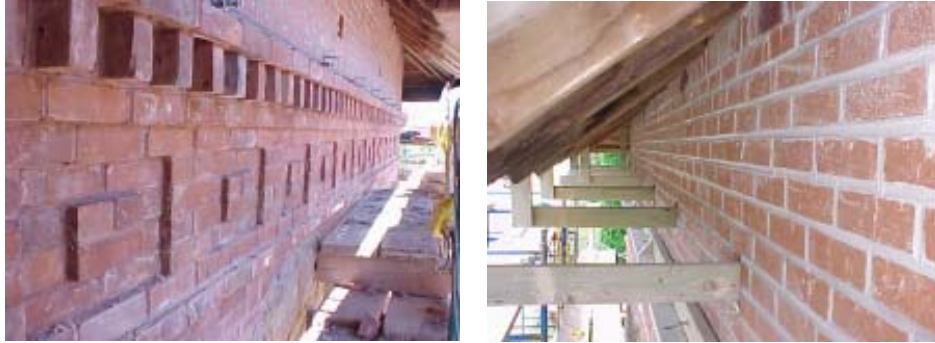
Figure 4. Reconstructed exterior wythe at (a) exposed frieze and (b) concealed area behind cornice.
