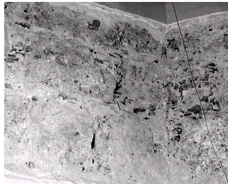
Figure 5. "Incoccio" probably used to widen the section of the pillars.
