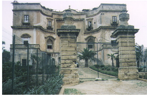
Figure 1. Frontal view of Villa Cattolica
