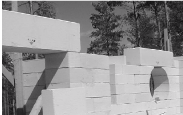
Figure 5 Lintel Bearing
