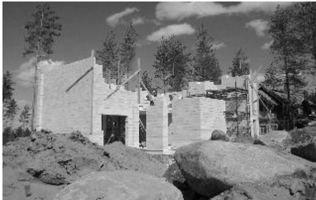
Figure 3 Solid Wall Construction
