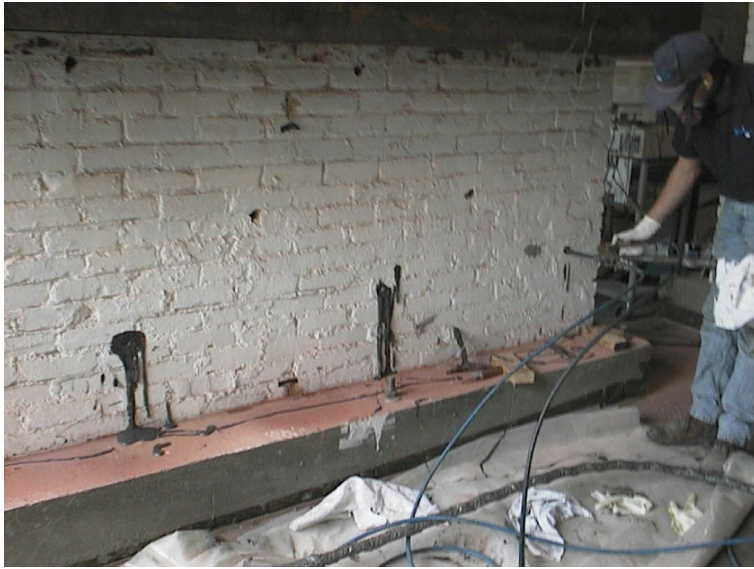
Figure 2: Pumping of Expansive Epoxy in the Wall
