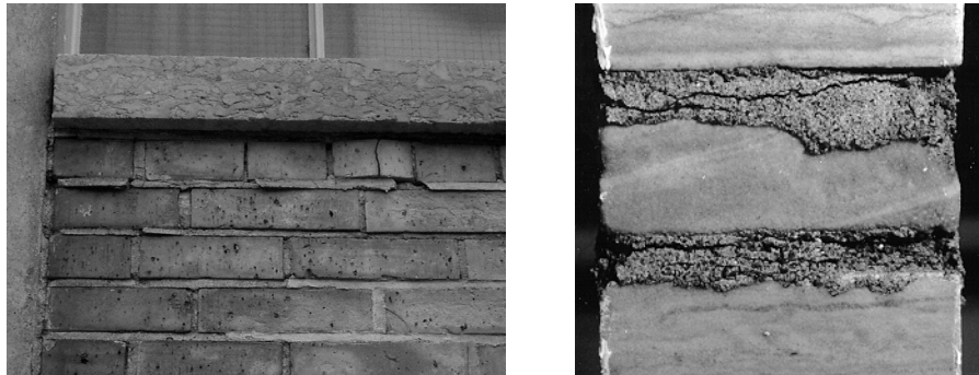
Figure 2. Frost damage
