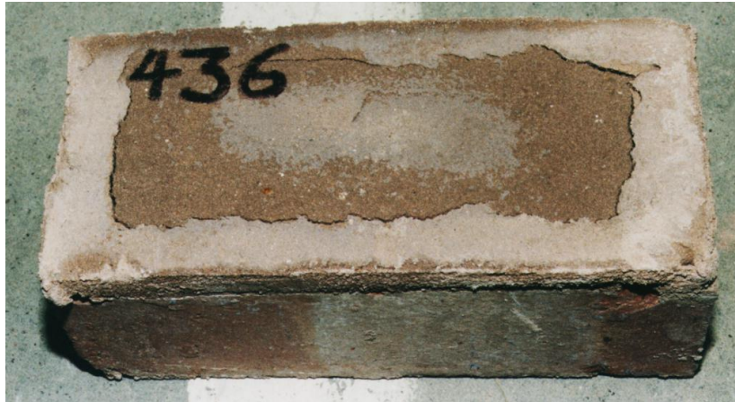
Figure 3. Differential shrinkage of the larger volume of shrinkable mortar in the frog of a semi-dry pressed brick causes debonding of the central area and retraction
