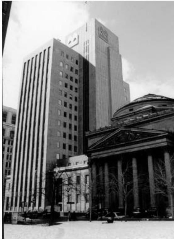
Fig 1 Head Office of the Bank of Montreal, Envelope restored in 1993
