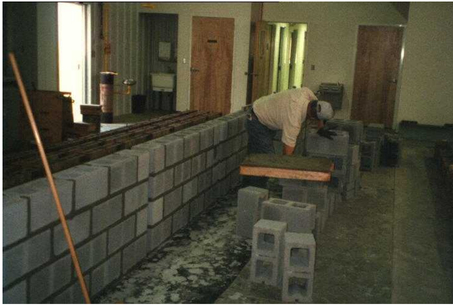
Fig. 2 - Hollow Concrete Masonry Walls Under Construction
