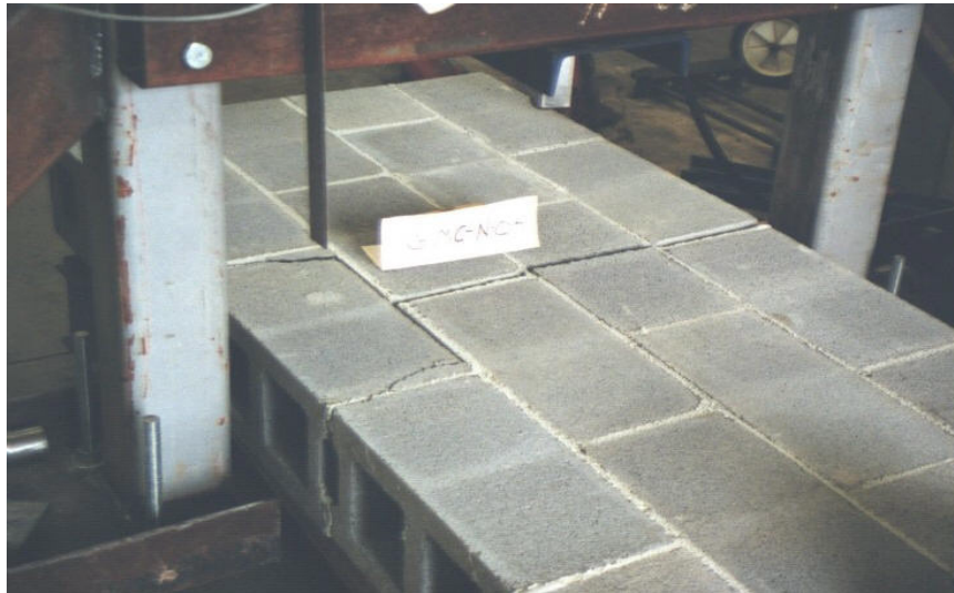
Fig. 8 - Failure Path Offset at Top Course – Hollow CMU Specimen
