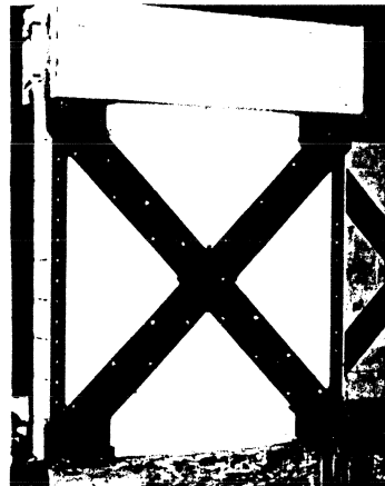
Figure 3 Retrofitting masonry wall
