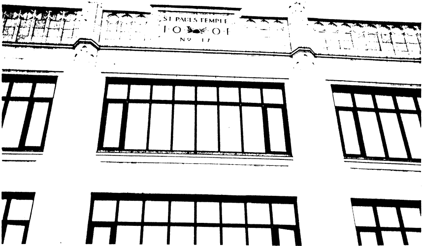
Photograph 7 - Repaired terra cotta
