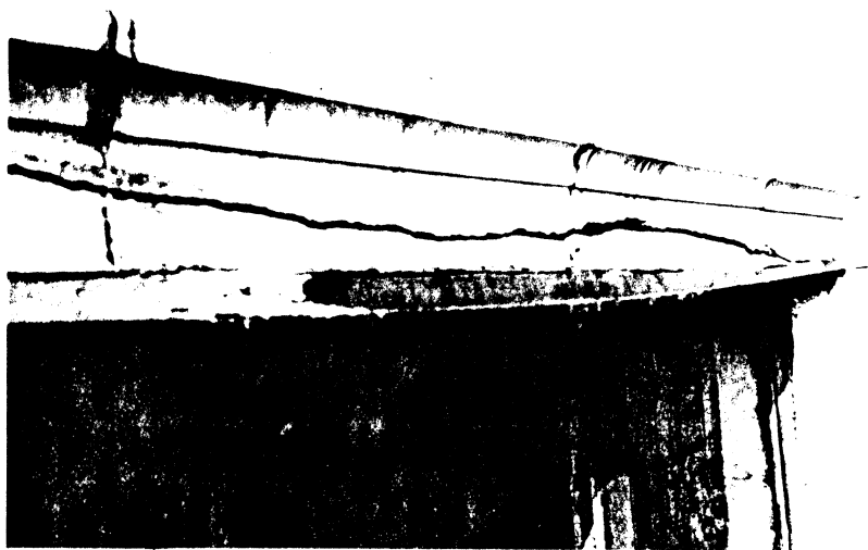
Photograph 2 - Broken terra cotta and head of window
