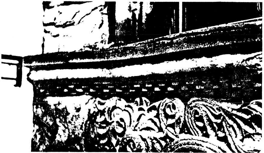
Photograph 3 - Deteriorated sill & scrollwork
