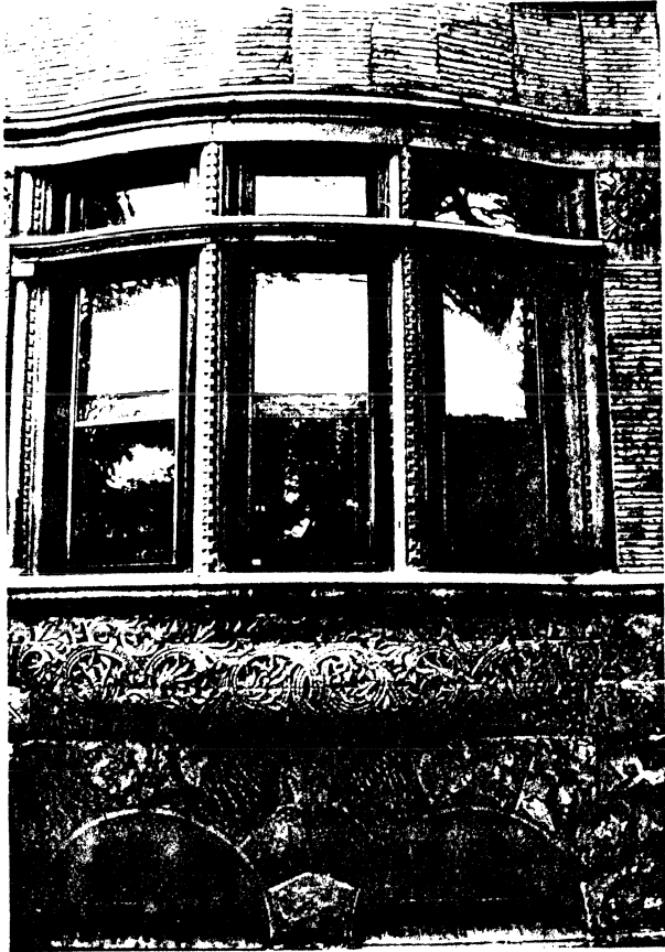
Photograph 6 - Restoration completed at lower level
