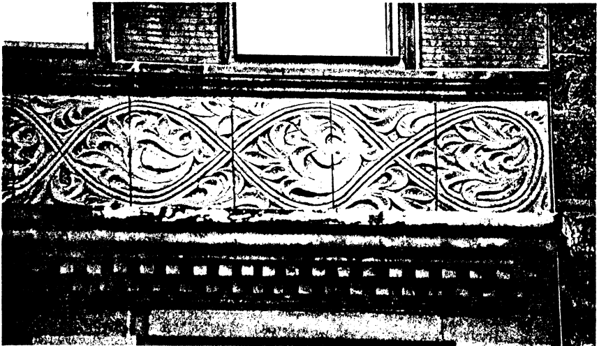
Photograph 5 - Restoration of scrollwork and details
