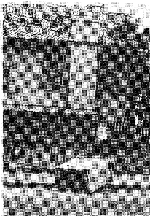
Figure 7: Large fallen unreinforced masonry chimney
