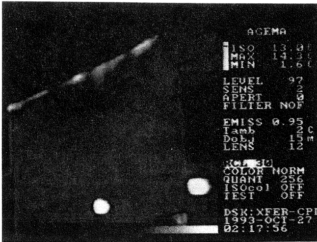
Photo 3 - Air Leakage at Roof/Wall Junction
