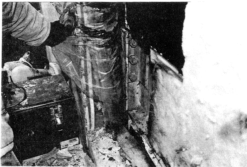
Photo 6 - Polyethylene Boots over Structural Steel/Block Interfaces
