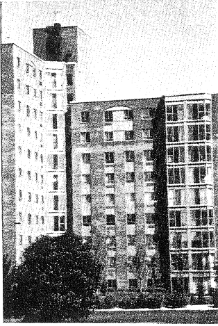
Fig. 1 S-W view of nine-storey apartment building
