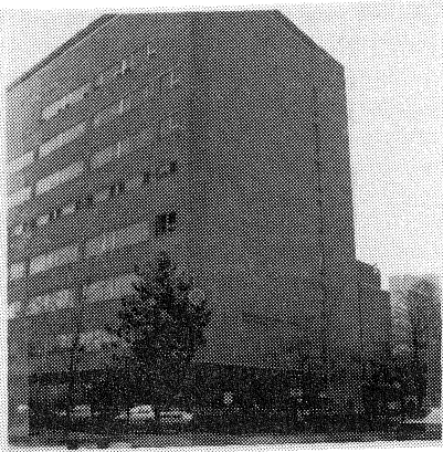
Fig 2. The Orthopaedic & Arthritic Hospital, Toronto - 1972 - Howard D. Vandewater, Architect, Toronto; SPF 38 mm (1½") thickness to masonry backup cavity wall. Exterior brick wall.
