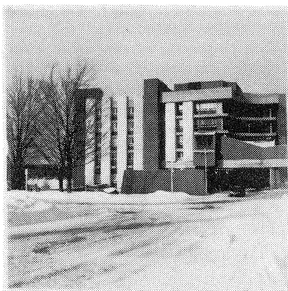
Fig 1. Health Sciences Centre, Penetanguishene - 1969 - Gilleland & Janiss Architects, Toronto; SPF 25 mm (1") thickness to masonry backup cavity wall. Exterior precast panel.
