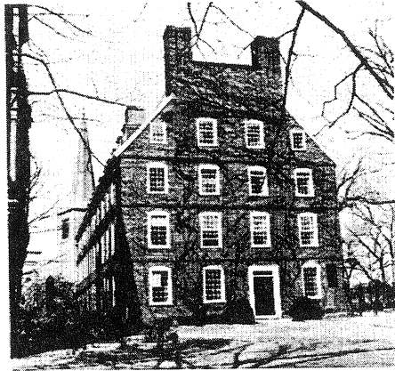
Fig. 1 Massachusetts Hall, Harvard University, built in 1720 with straight lime-sand mortar. The mortar has never been replaced, repaired, or tuckpointed. (Boynton et al. 1964)
