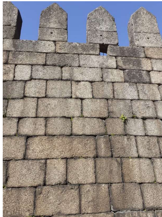
Figure 1: Masonry pattern using regular blocks for the historic perimeter wall of Guimarães, Portugal
