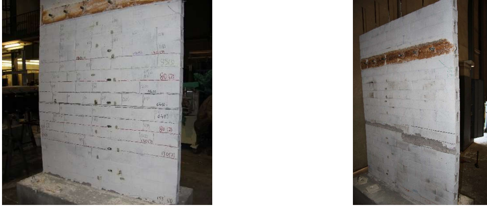
(a) (b) Figure 4: Typical cracking pattern: (a) rear face; (b) front face
