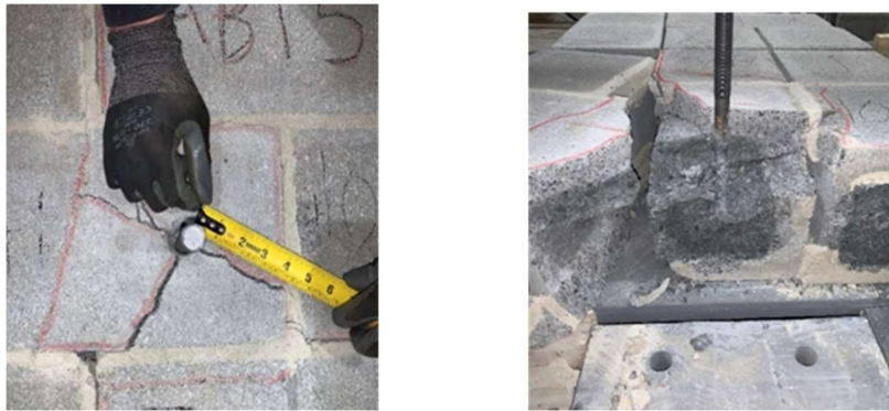
Figure 4: a) Radial cracks AABT5-1 b) Break out cone and splitting along the mortar
