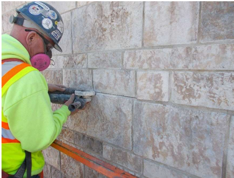
Figure 3: Mortar Joint Removal Using a Diamond-Tipped Cutting Wheel
