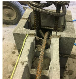
b) Bond beam detail
