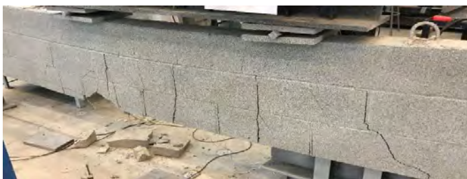
Figure 9: Failure mode of specimen F-8S
