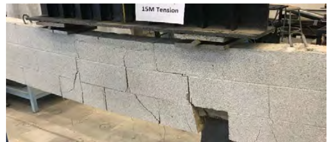
Figure 7: Failure mode of specimen F-10M
