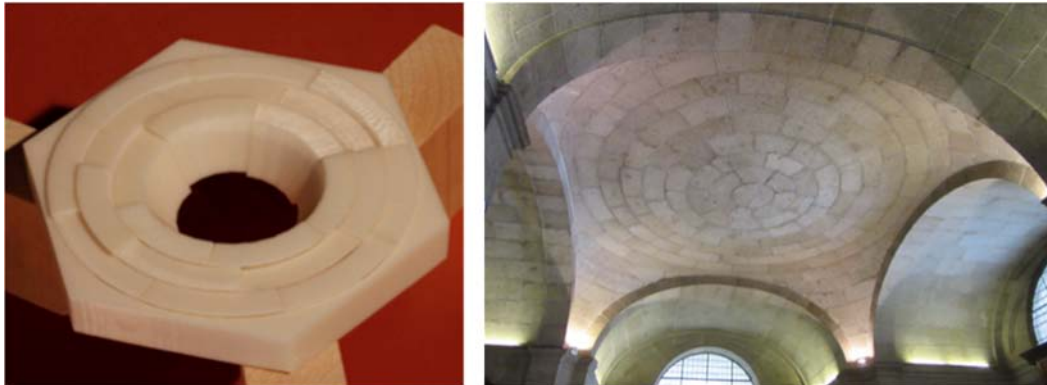
Figure 8: 3d Printed Plastic Floordome (150mm dia.) and Herrera's Vault (7.81m dia)
