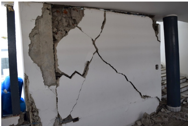
a) Termination without a frame column
