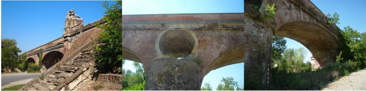
Figure 2: Taro bridge (Ponte Paro), Parma, Italy
