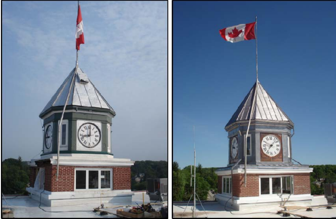
Figure 12: Original (left), Restored (right)
