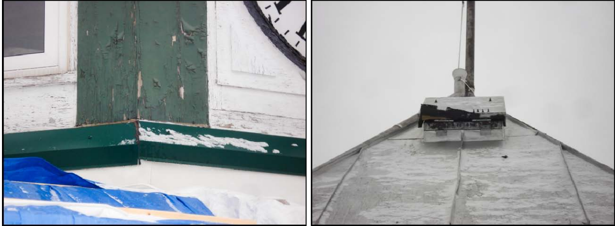
Figure 9: Sources of Water Infiltration
