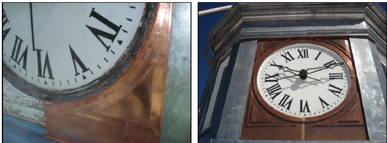
Figure 11: Copper Re-Cladding Underway (left), Tower Re-Cladding Complete (right)
