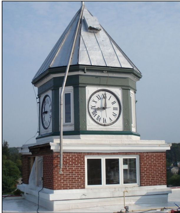
Figure 2: Existing Condition of the Clock Tower (August 19, 2013)
