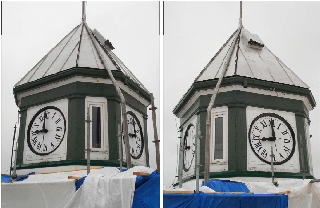
Figure 8: Tower During Construction (November 18, 2013)
