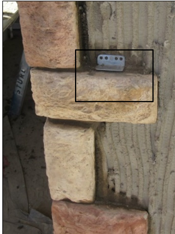
Figure 7: L-plate used as a brick tie
