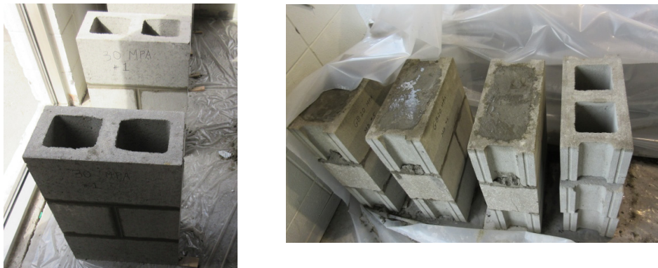
Figure 1: Constructed Hollow and Grouted Prisms
