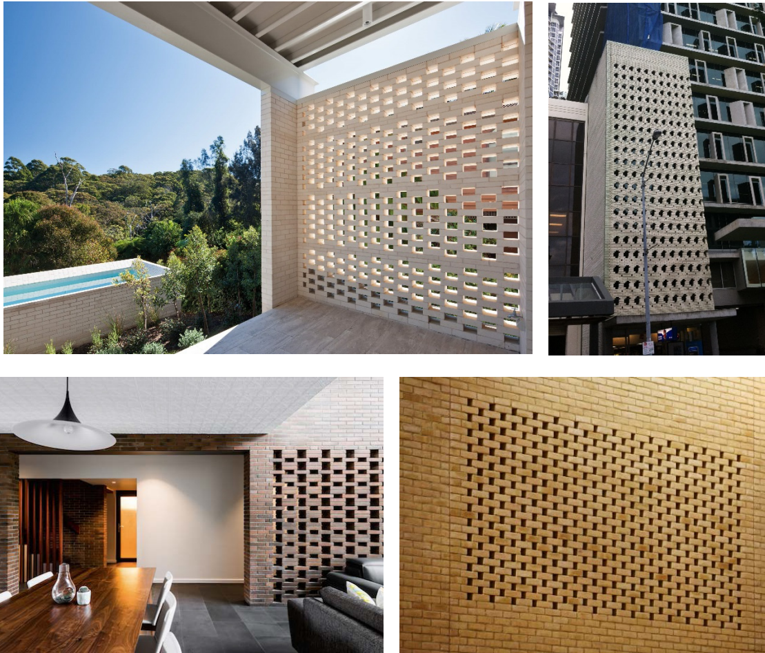
Figure 1: Examples of Lattice Masonry Construction, also known as “Hit and Miss Brickwork” (photographs supplied by Think Brick Australia)
