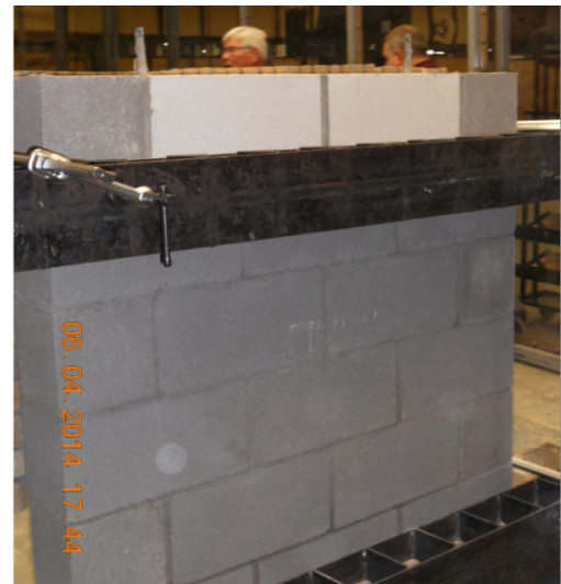
Figure 14: Back of CMU Wall on Specimen 2 After All Missile Strikes
