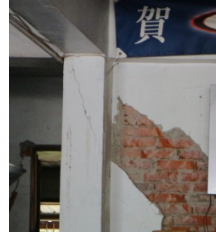
(a) Damaged masonry panel with eccentric door opening (b) Shear crack on the column
