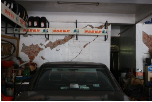
(a) Damaged masonry panel with eccentric door opening (b) Shear crack on the column
