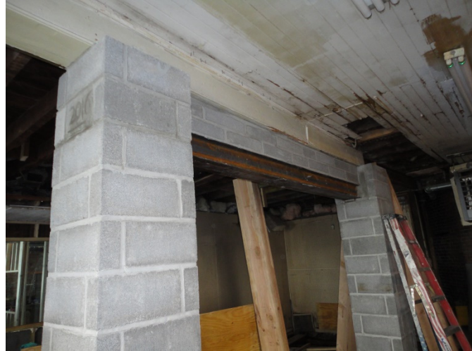
Figure 15: Jacking Beam/Permanent Support
