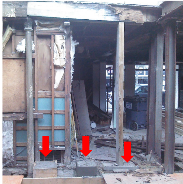
Figure 18: Jacking Locations
