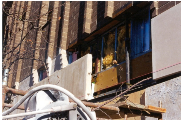
Figure 12: Shoring during Rebuild
