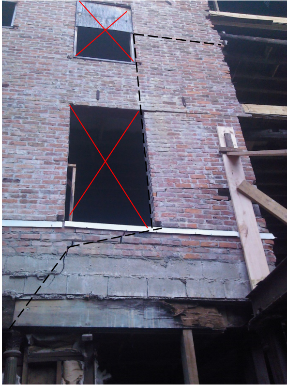
Figure 17: Cracked Wall
