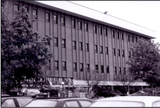
Figure 9: Four-story Steel-framed Office Building
