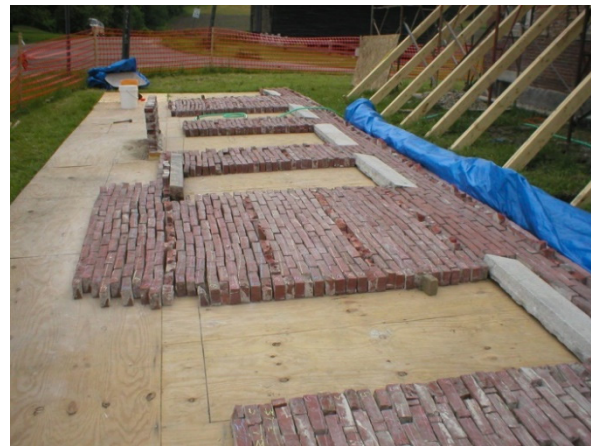
Figure 8: Exterior Leaf and Headers
