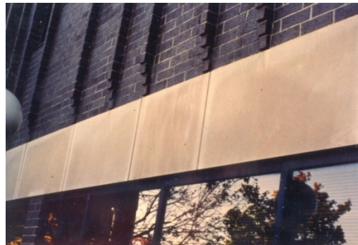
Figure 10: Stone Trim at Bottom of Brick Veneer
