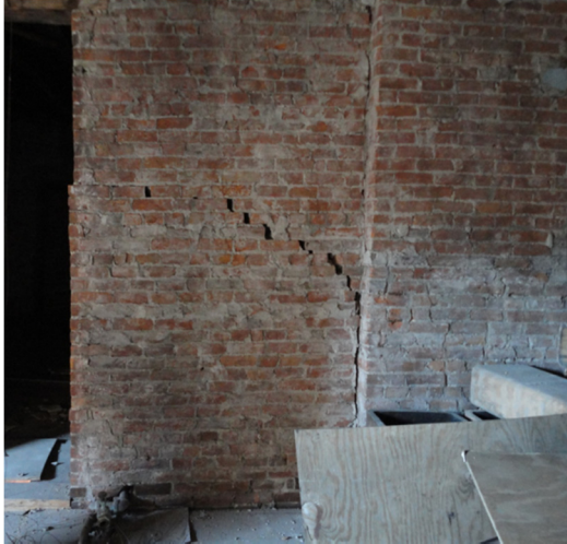
Figure 14: Cracked Wall
