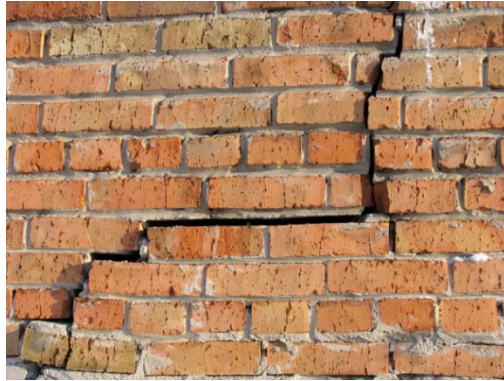
Figure 3: Masonry Cracks
