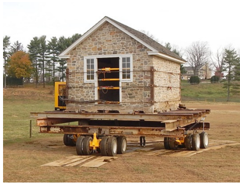
Figure 1: Moving a Masonry Building (Courtesy Of Buckingham Structural Moving Equipment, Bernville, PA)
