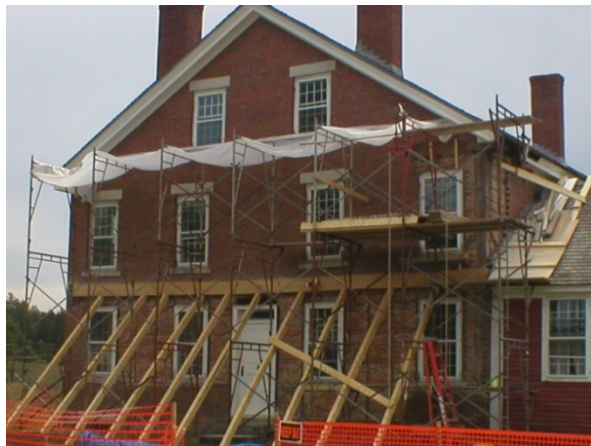
Figure 7: Shoring Installed
