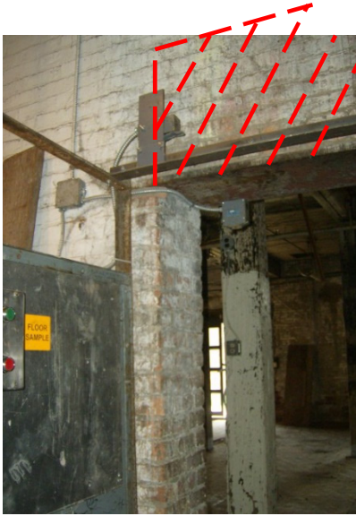
Figure 4: Existing Opening to be Enlarged Vertically
