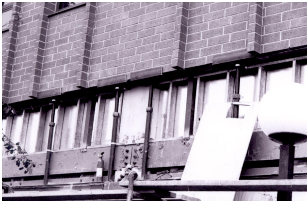
Figure 11: Shoring after Panel Removal
