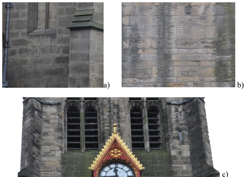
Figure 9: Typologies of Masonry: a) Ground Level, Typology A, b) Under the Clock Level, Typology B, c) Over the Clock Level, Typology C
