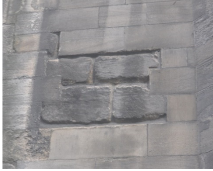
Figure 10: The Original and New Stone Block Added After 19 th Century Restorations
