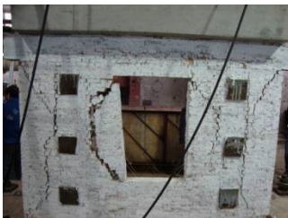
(a) Crack of Masonry Wall
