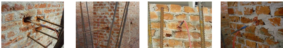
Figure 4: Construction of connection joint
