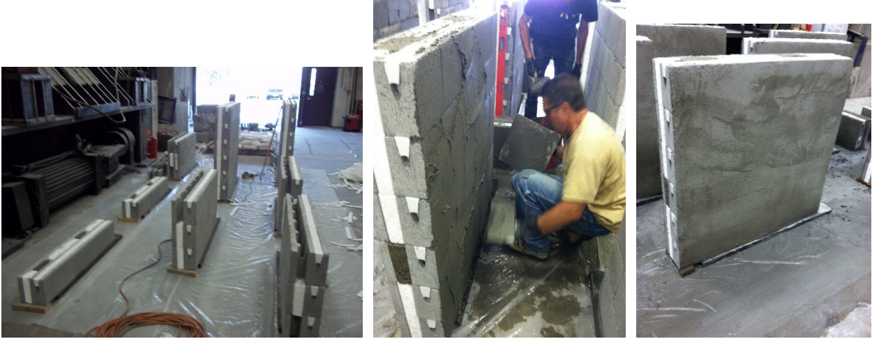
(a) Blocks Being Laid. (b) Application of Surface Coating (c) Curing
