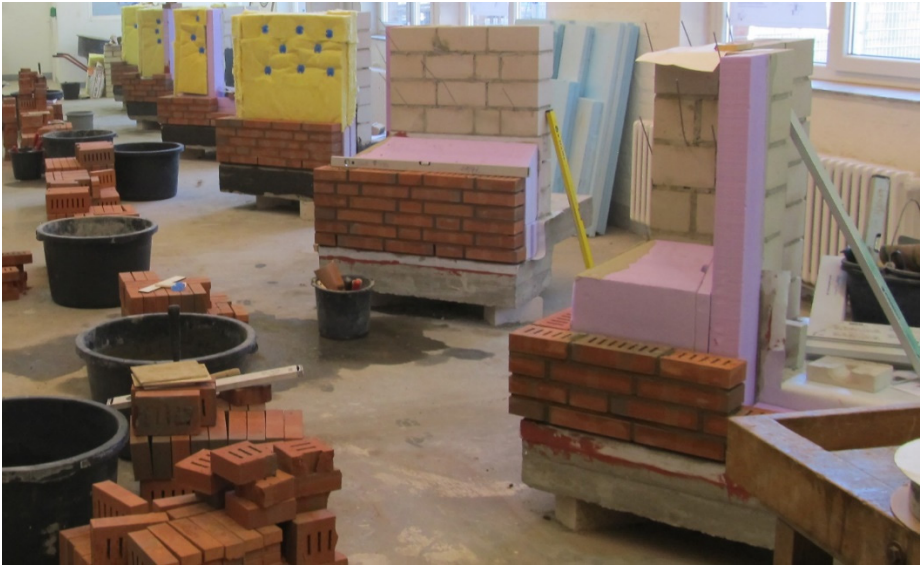
Figure 7: Test walls to investigate the watertight construction of windows and ground-level door openings considering corners and edges under construction
