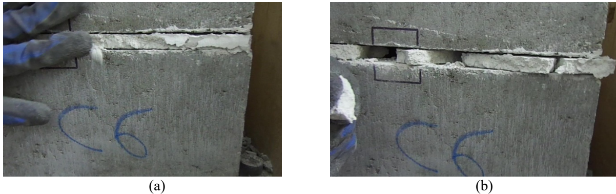
Figure 5: Aspect of the mortar joint of prism W6 after the failure
