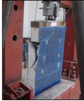
Figure 2: Tested wall retrofitted with CFRP and corresponding to “Compressive test 3” in Table 2 (Chagas and Moita [7])
