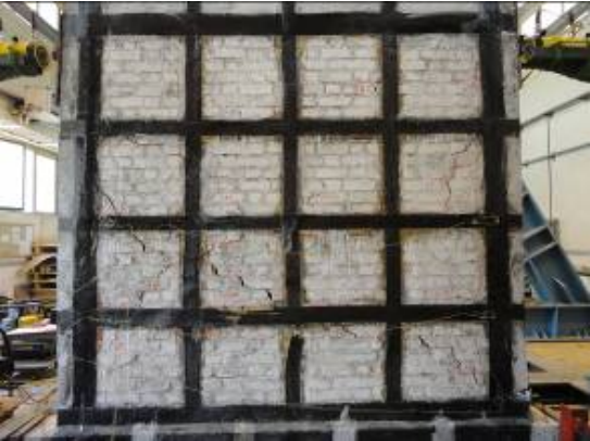
Figure 9: Crack Pattern of the Retrofitted Wall with CFRP
