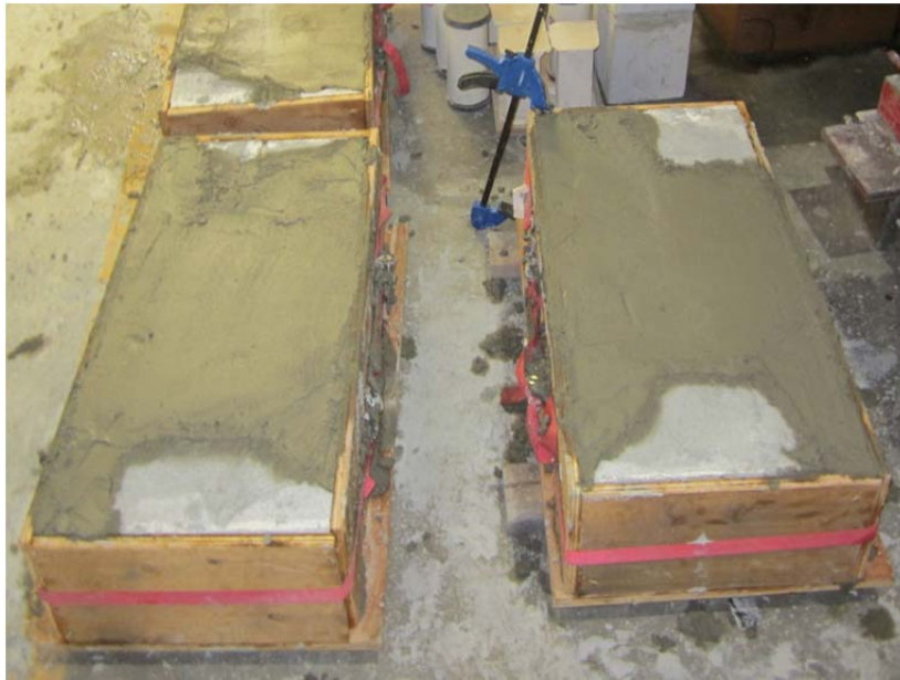
(b) Prisms Shown After Completion of Repair Grouting
