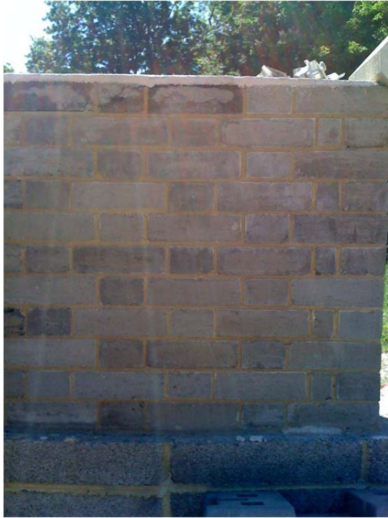
Figure 3: Masonry test panel constructed at Poundbury
