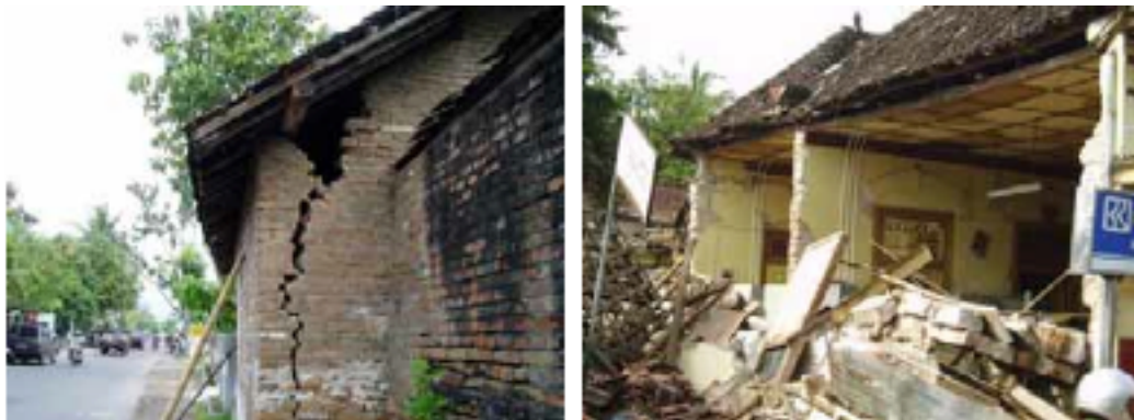
Figure 2: Half brick thick masonry buildings without reinforcements [13]
