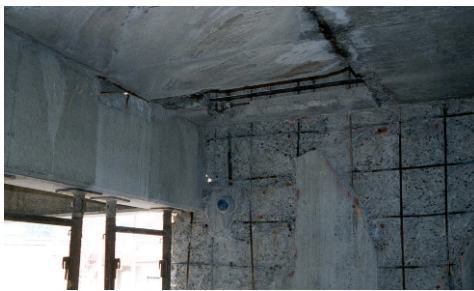
(b) Corrosion Problem in RC Structures
