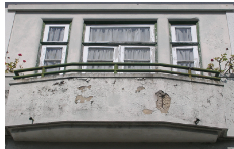
(b) Corrosion Problem in RC Structures
