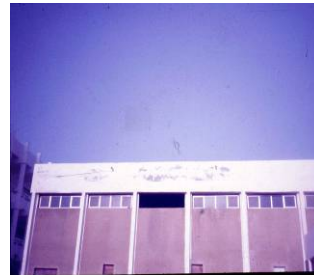
(a) Spalling and Cracking of the Building Envelope
