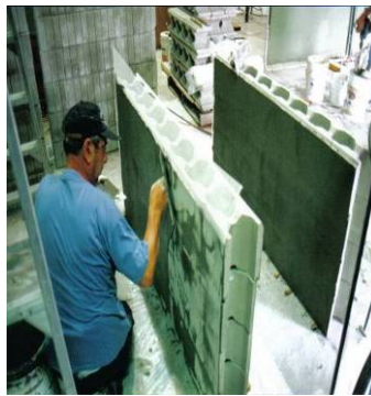
(b) Surface plastering
