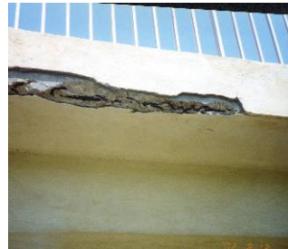
(a) Spalling and Cracking of the Building Envelope
