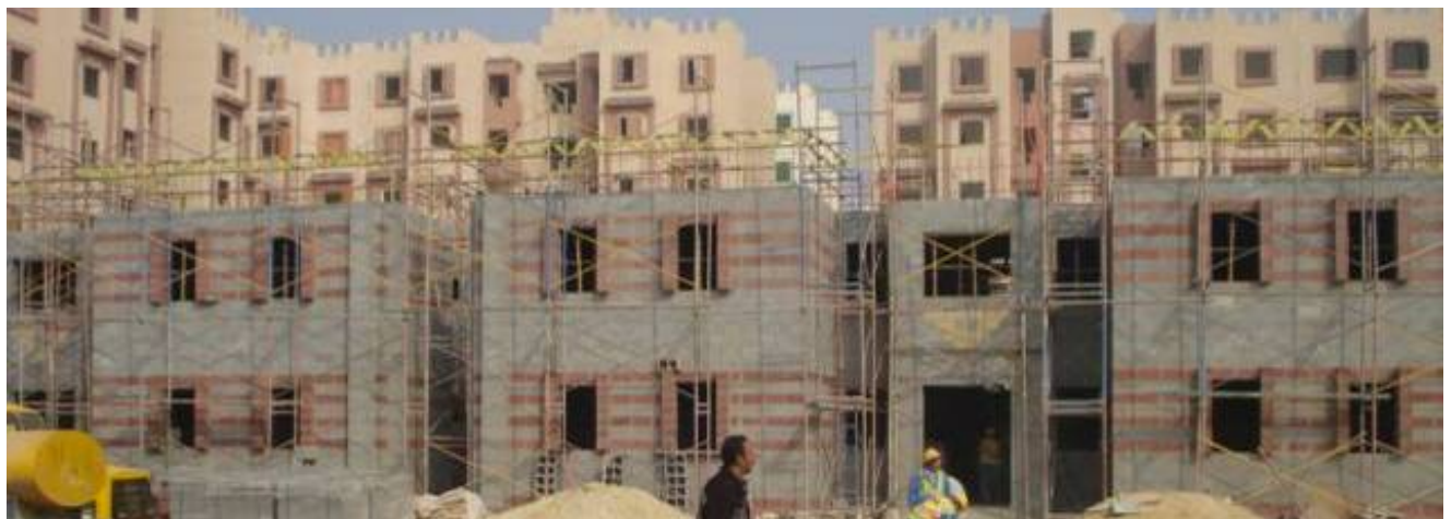
Figure 4: Loadbearing Masonry Buildings under Construction
