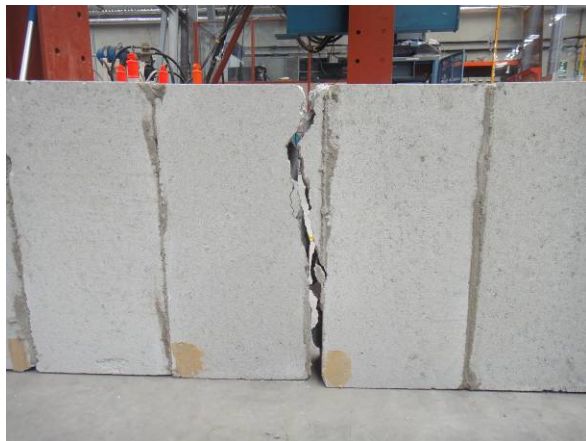
(c) Beam (partial block failure)
