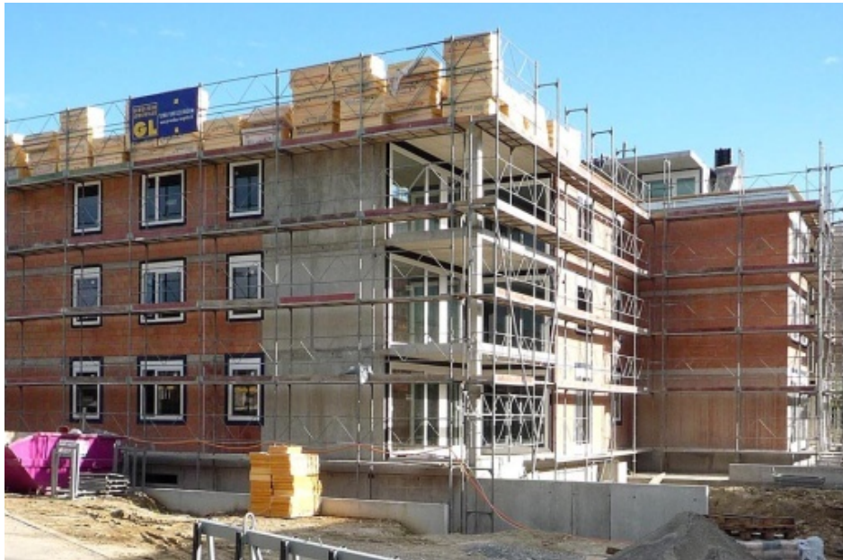
Figure 1: Typical mixed RC-URM wall structure (Photo: T. Wenk).
