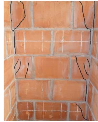
b) Cracking patterns of clay specimens
