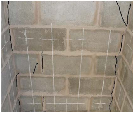
a) Cracking patterns of concrete specimens
